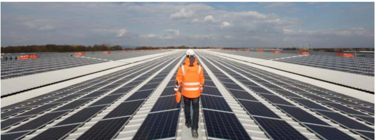
Solarcentury roofs: combined heat and power for a housing association, solar electric for a superstore.
